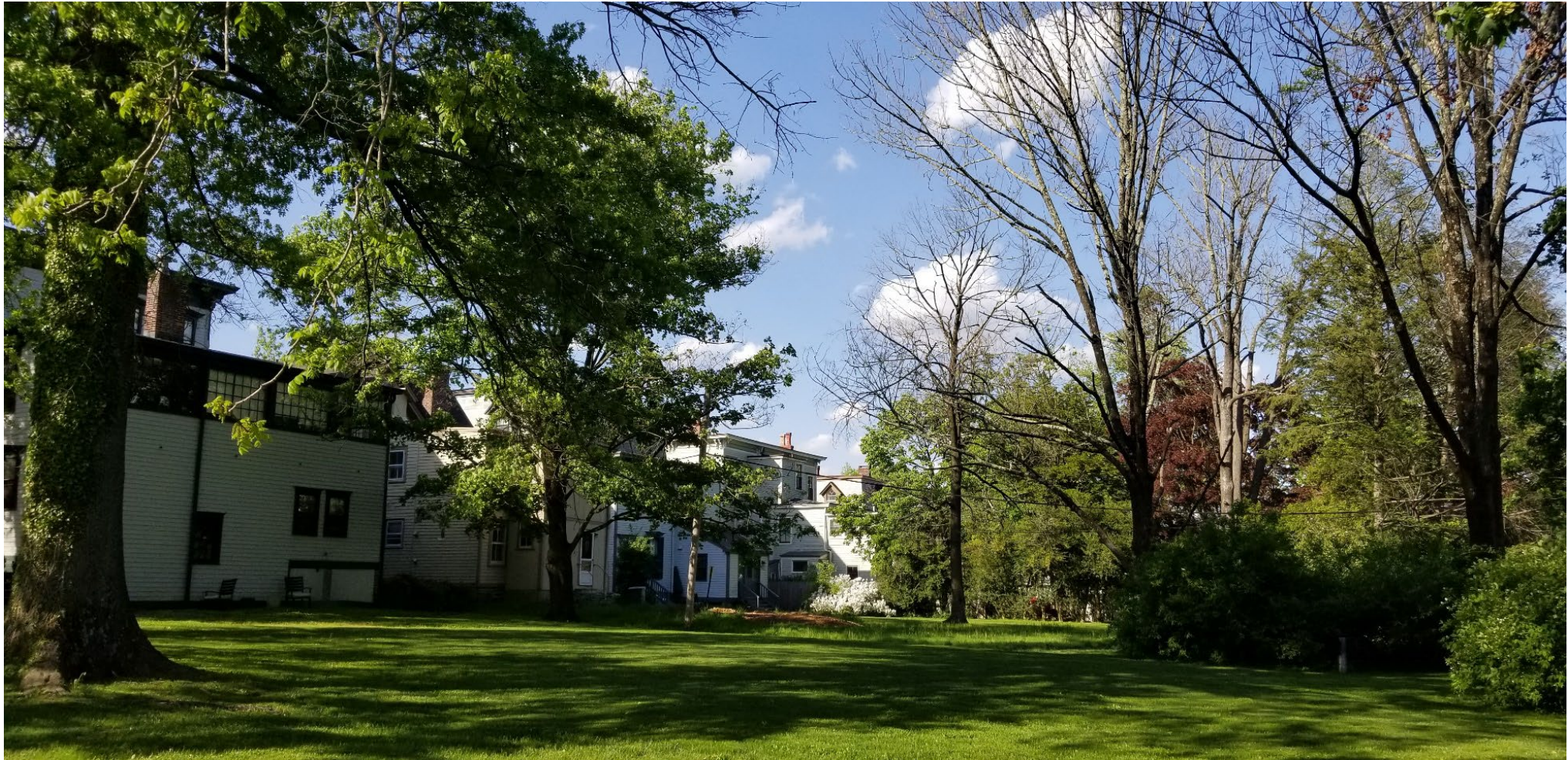
Looking from Alexander Street at rear elevations of #16, #22 Dickinson Street and others
