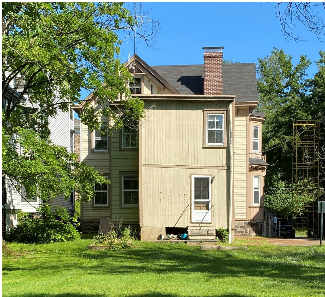
SouthEast Elevation - Rear
